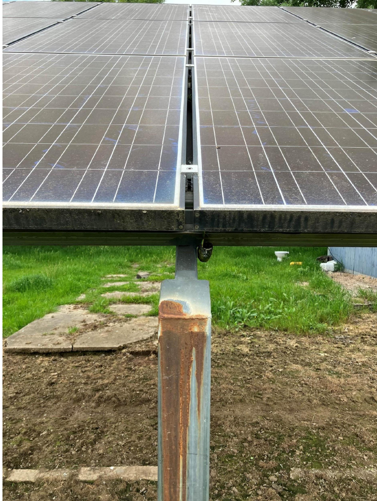
Run off corroding galvanised post
