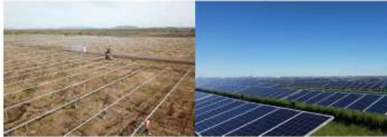
Figure 4 Pile driven steel posts with tracker assemblies
