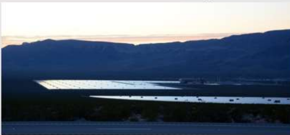
Figure 5.2-1. Black PV Panels at CM 1 and 2 Facilities Appear White When Low-Angle Sunlight is Reflected from the Panels (Background), and the PCU's look black.
