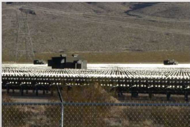
Figure 6.2-4, Reflections from Multiple Regularly-Spaced Components in the SSN PV Panel Array.
