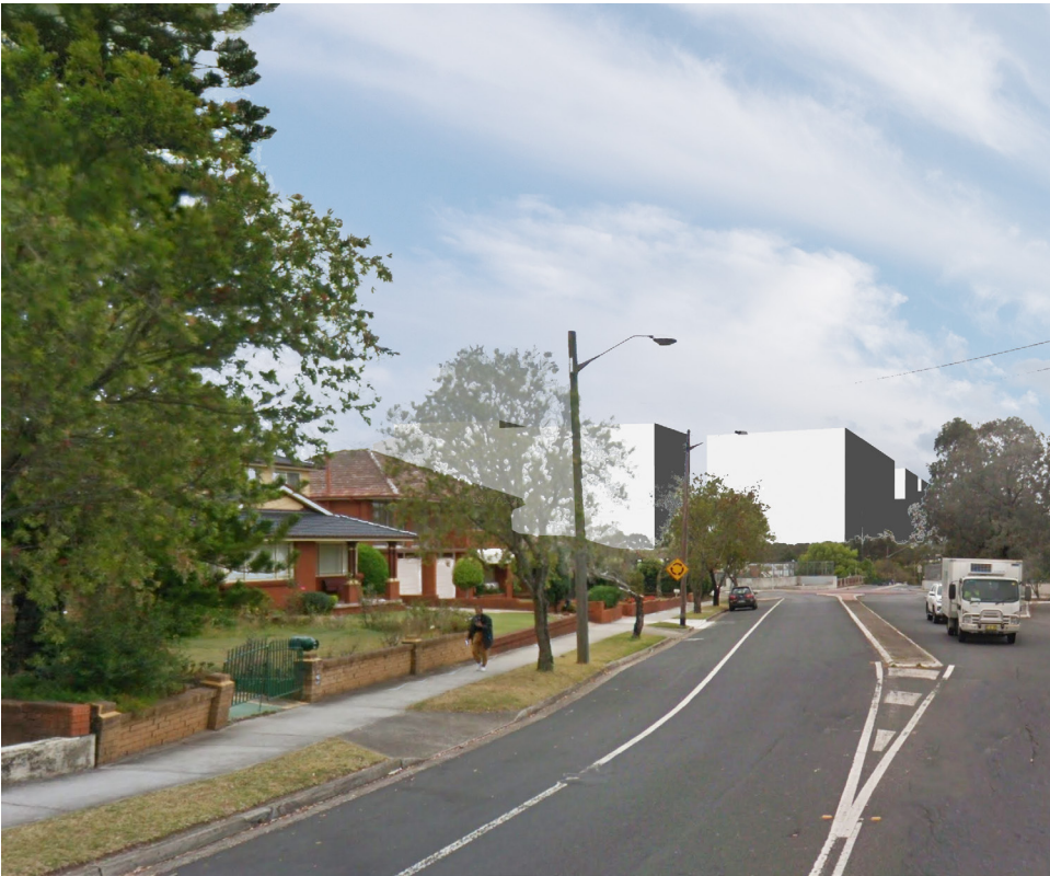
Ⓐ Fig. 1 View from Auburn Rd
