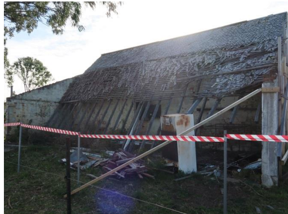
PICTURE 14 – THE REAR OF THE FORMER COACH HOUSE HAS COLLAPSED AND THE TIMBER SHINGLED ROOF IS EXPOSED
