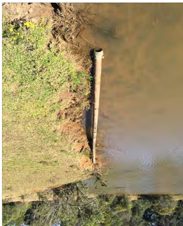
Photograph 2 - Dam bank and loose pipe from pump system
