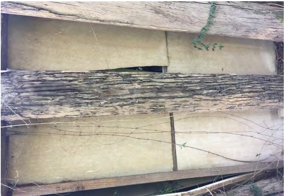
Photo 4 - Suspected ACM eaves visible in former homestead structure
