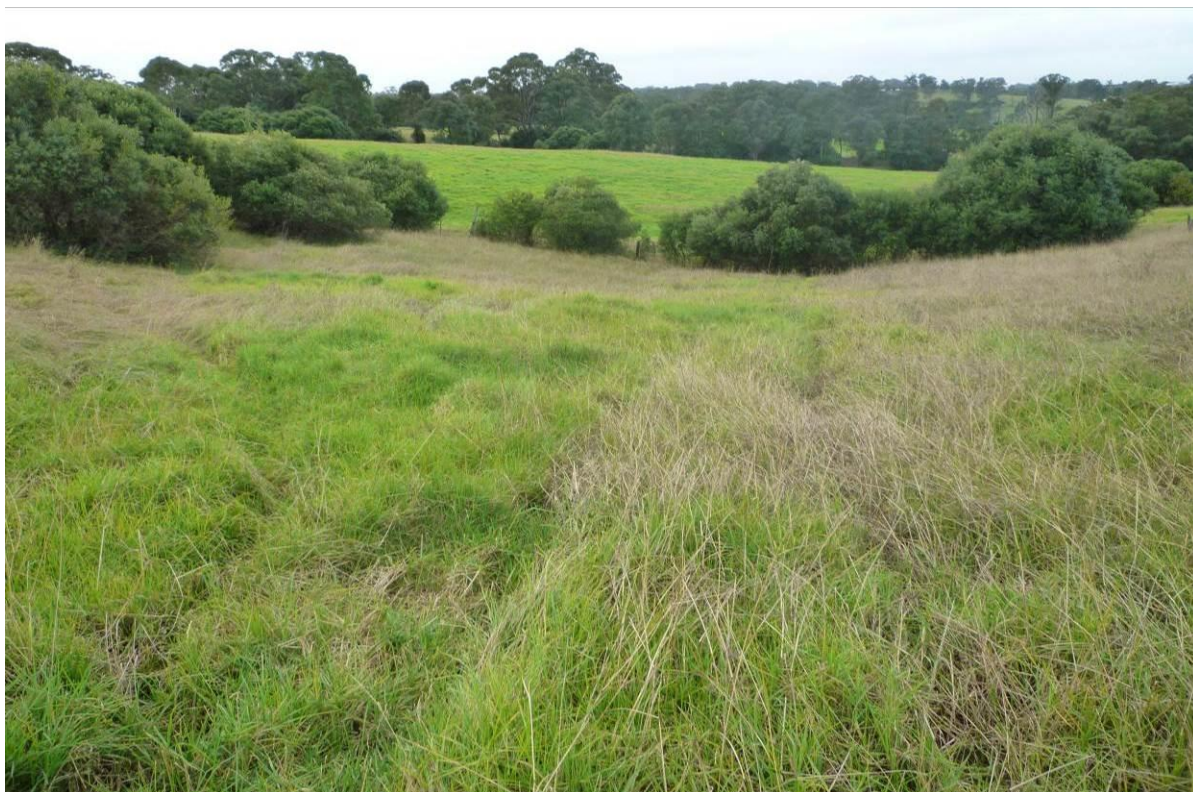
Photo 35 – Drainage line 14, grassed swale with no evidence of drainage < 12 hours after heavy rain
