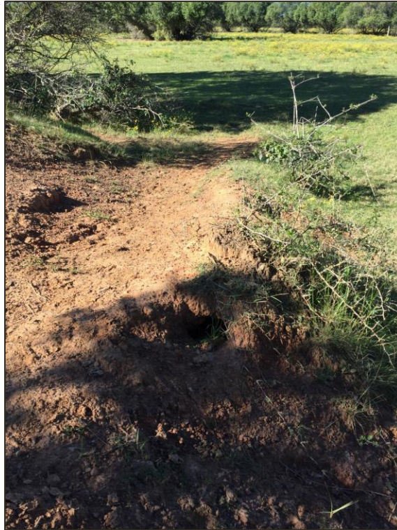
Burrow at south-eastern end of downstream shoulder
