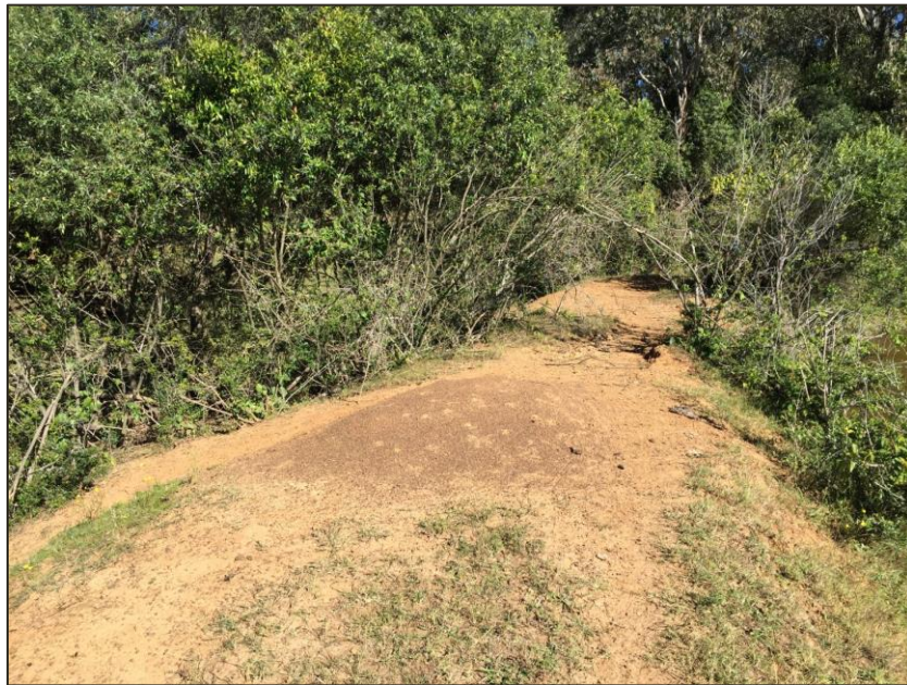
Ant hill on Dam 5 embankment crest
