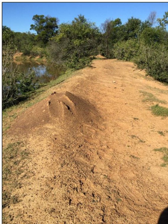
Ant hill at north-western end of Dam 7 embankment
