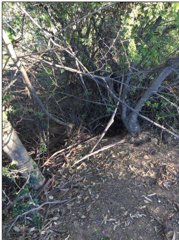
Burrows in downstream shoulder of Dam 10 embankment
