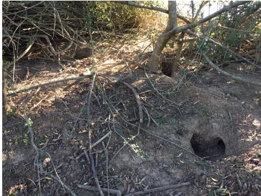
Burrows in downstream shoulder of Dam 4 embankment
