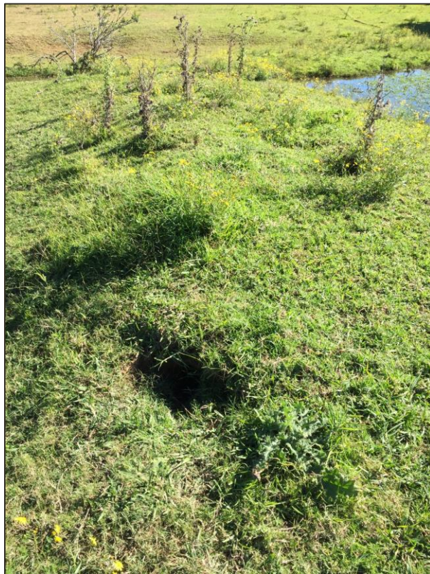
Burrow at western end of Dam 6 embankment
