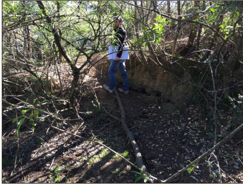
Sub-vertical toe along downstream shoulder of Dam 7 embankment
