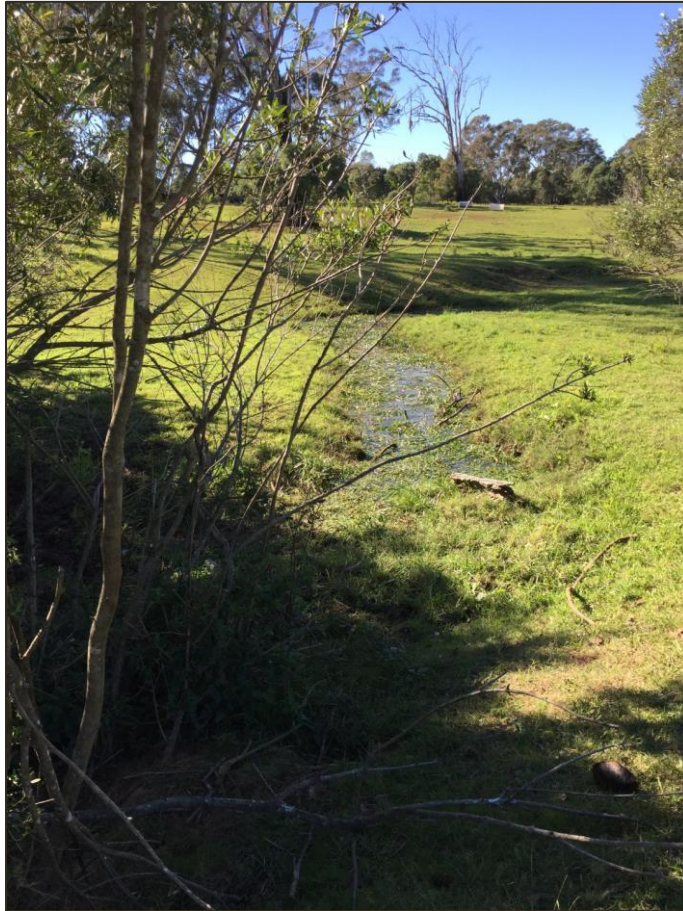
Stagnant water in creek beyond downstream toe of Dam 4 embankment
