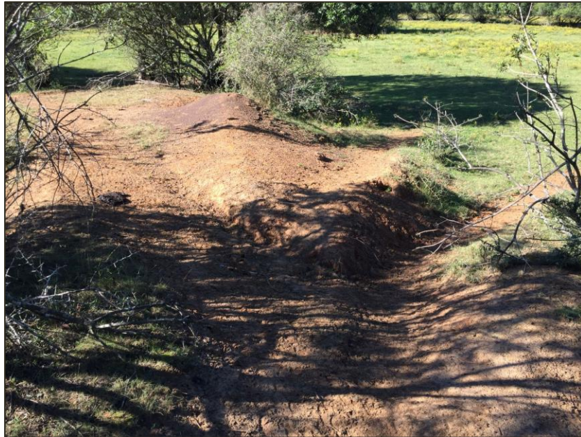
Erosion features on downstream shoulder of Dam 7 embankment
