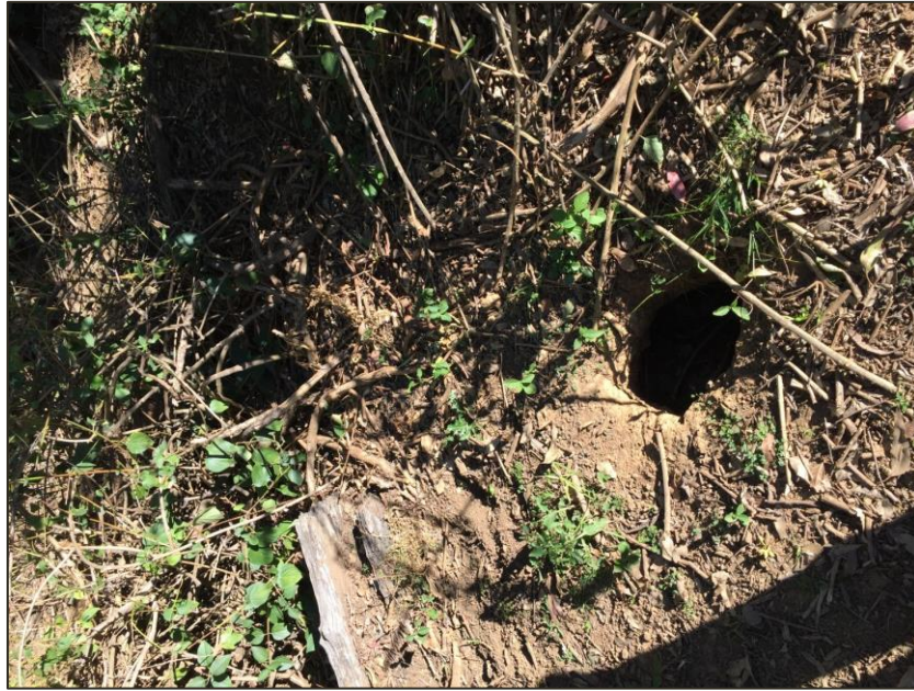
Burrow in Dam 8 embankment
