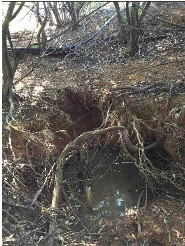
Deeply incised erosion feature at downstream toe of Dam 8 embankment
