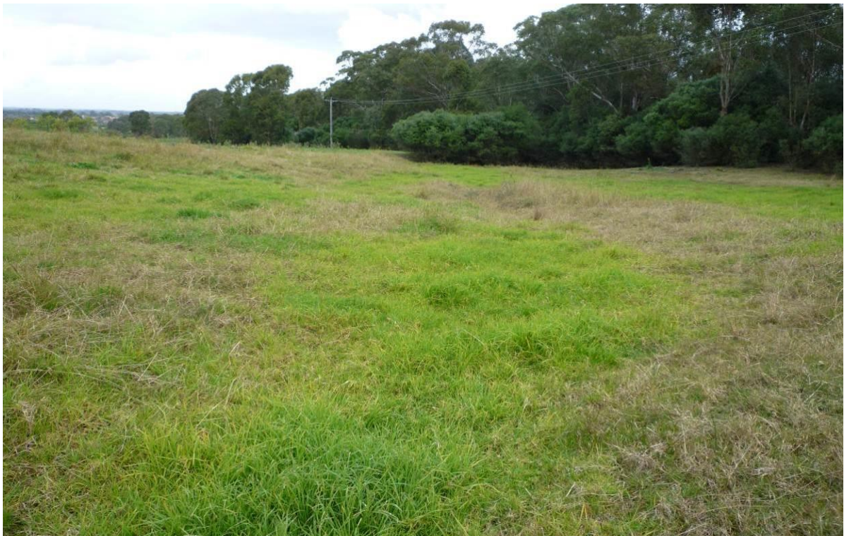
Photo 24 – Drainage line 11, grassed swale with small dam at head no evidence of drainage < 12 hours after heavy rains
