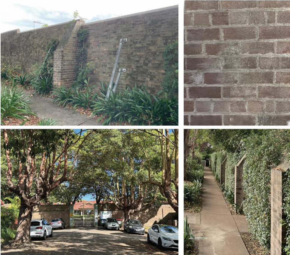
Existing heritage boundary wall
