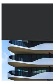
Fixed vertical metal fins balustrades with top rail in powdercoat finish to match **Dulux Monument**
