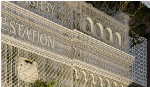
Material - Reinterpret original details through a woven wire mesh as a distinctly new material to reference memory.
