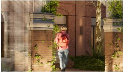
Retention - Salvage materials and form new capitals to reconstruct piers
