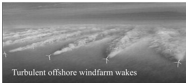
**Figure 1.** Turbulent moisture-laden wakes in an offshore windfarm near Denmark.
