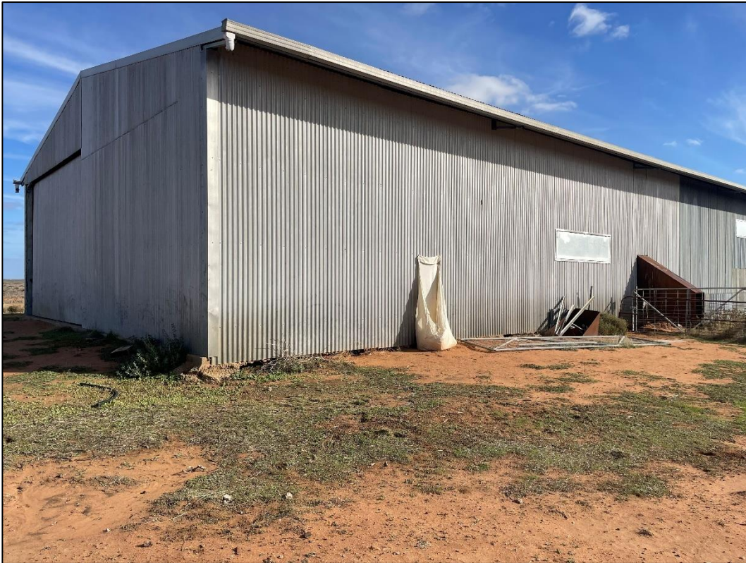
Plate 7: Built structures within the Project Area but outside of the Disturbance Footprint include farm sheds.
