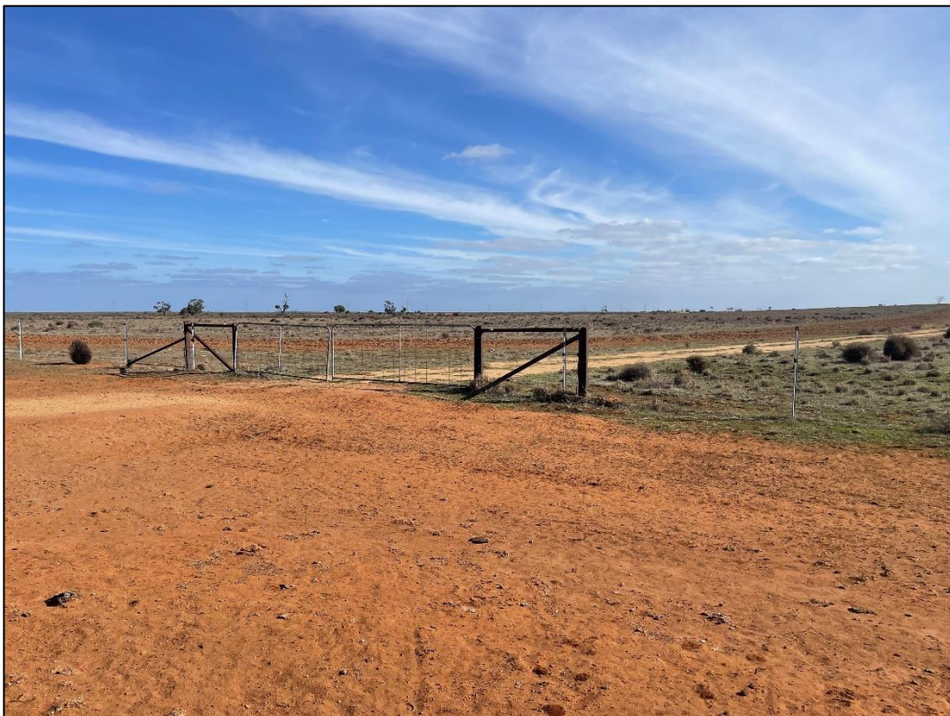
Plate 6: Built structures within the Disturbance Footprint are generally limited to gates and livestock fencing.
