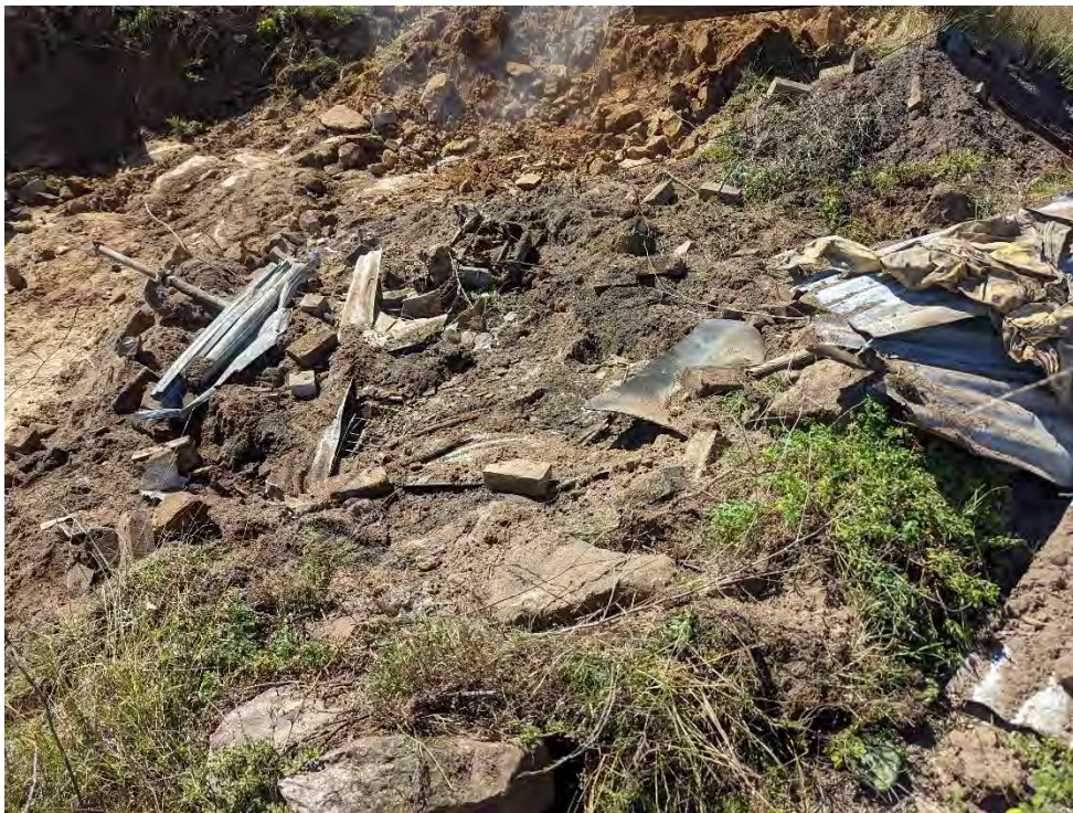
Photo 23: Location 25 – Cement sheeting and miscellaneous debris present within the rubbish dump, during asbestos and mixed waste removal work
