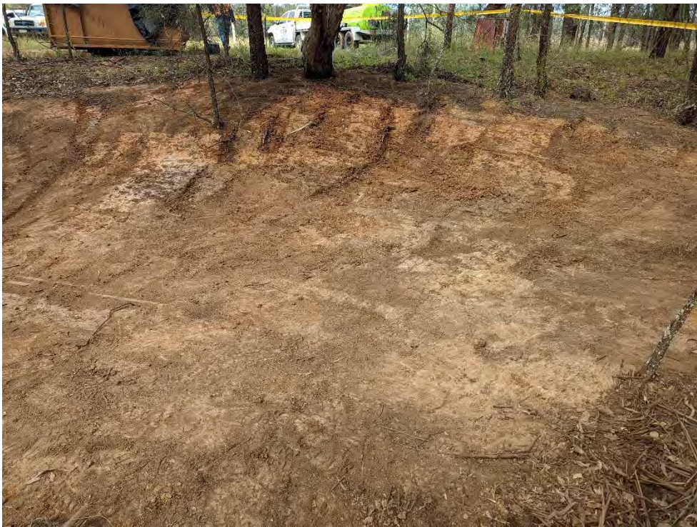
Photo 28: Dog Track – Visible and accessible residual soil surfaces following the completion of the current scope of asbestos removal work
