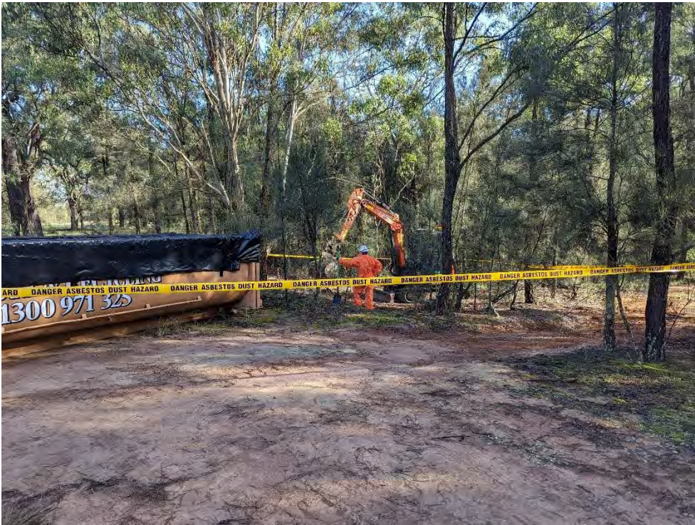
Photo 27: Dog Track – Asbestos removal works undertaken by excavation and offsite disposal of impacted topsoils
