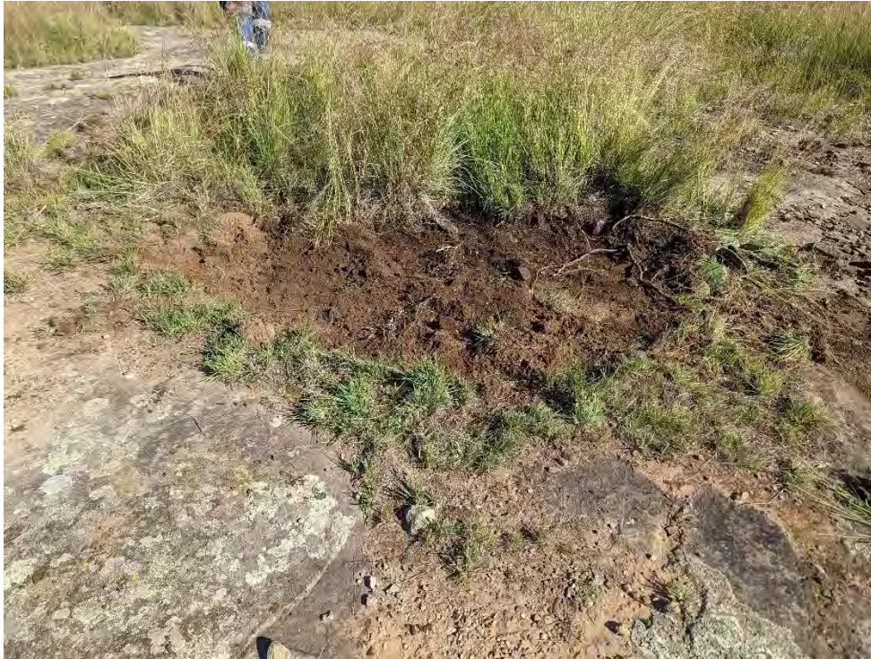
Photo 20: Location 24 – Visible and accessible residual soil surfaces and rock surfaces following the completion of hen-pick asbestos removal works
