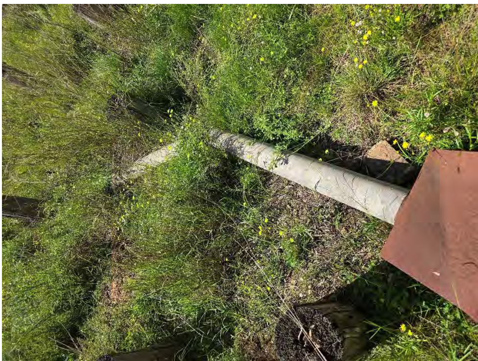
Photo 29: Bra Gate – Asbestos conduit present within structure footprint prior to removal work
