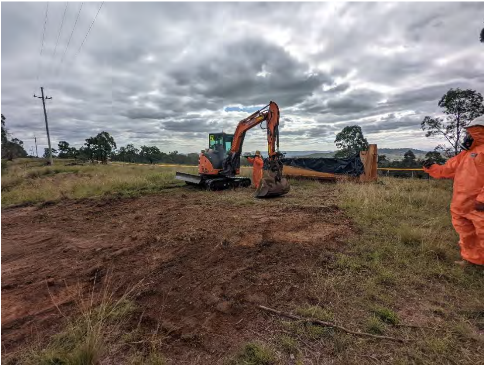
Photo 6: Location 14 – Wash-down of excavator following the completion of asbestos contaminated soil excavation work
