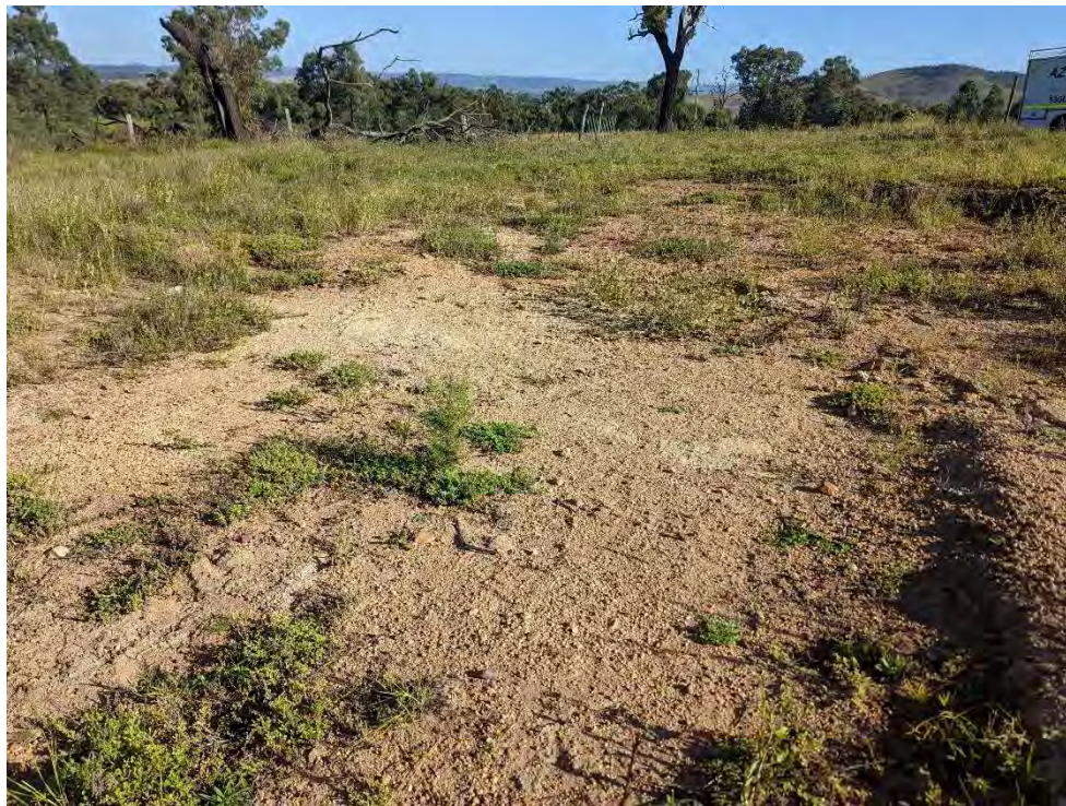
Photo 16: Location 22 – Visible and accessible residual soil surfaces following the completion of hen-pick asbestos removal works
