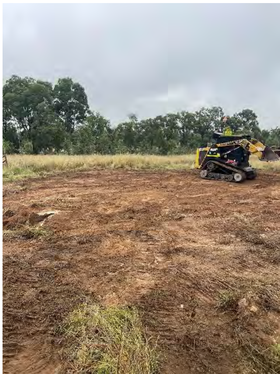
Photo 24: Location 25 – Site surface reinstatement following the completion of asbestos and mixed waste removal works from the rubbish dump
