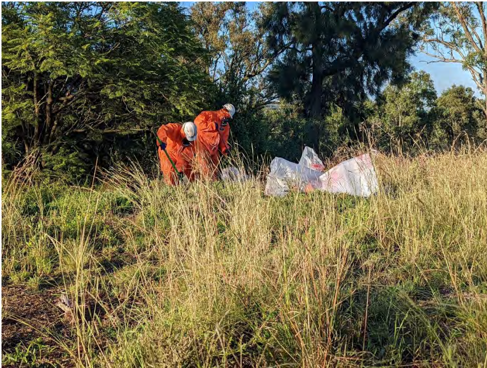
Photo 4: Location 14 – Asbestos removal works by hen-picking debris
