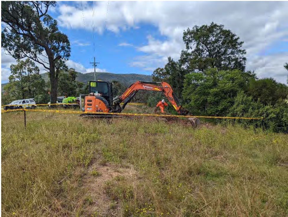
Photo 5: Location 14 – Asbestos removal works by excavation of topsoil into onsite skip bin
