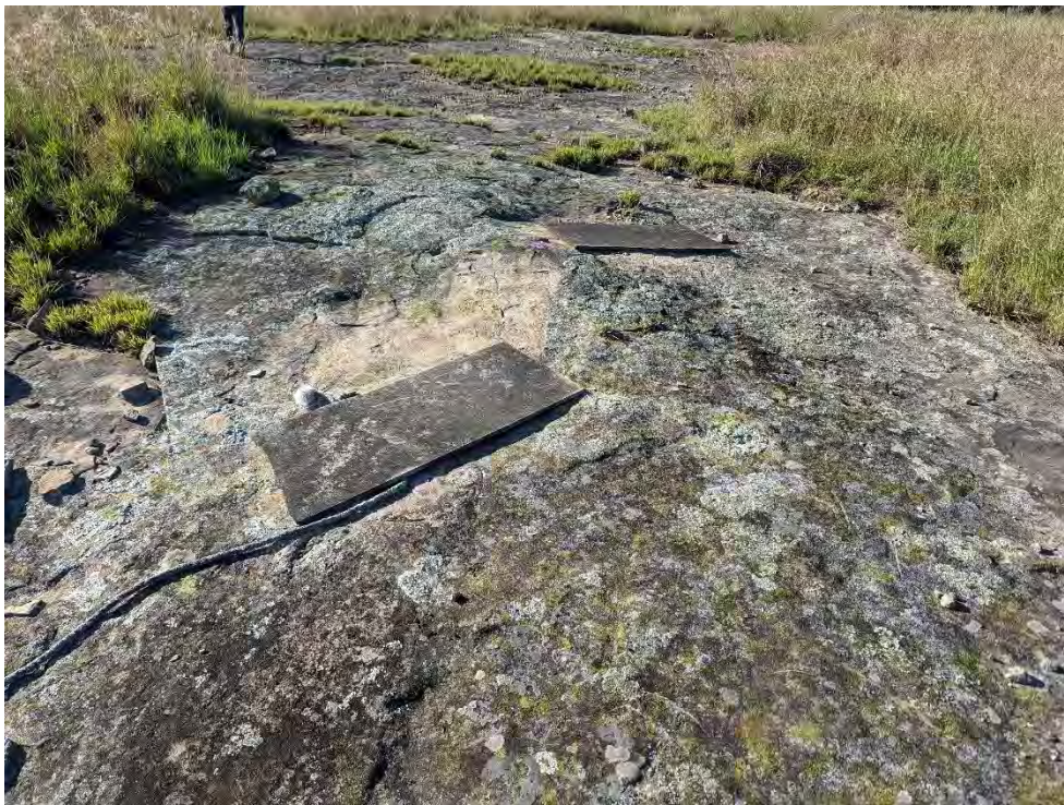
Photo 17: Location 24 – Large cement sheets present on rocky outcrop prior to asbestos removal work
