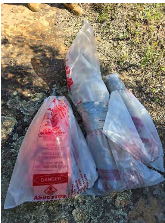
Photo 30: Bra Gate & Location 16 – Bulk asbestos waste and used PPE bagged during asbestos removal work
