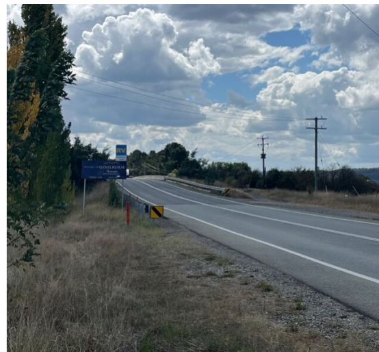
Figure 4 – Locality tour, view of the bridge crossing of the Mulwaree River from the south of the bridge
