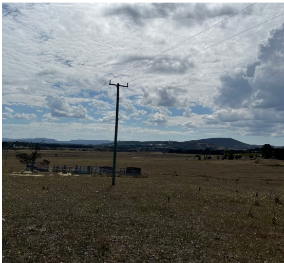
Figure 3 – Location 2, existing infrastructure on the Site
