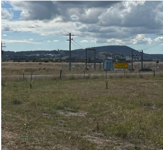
Figure 1 – Location 1, view of existing substation north of Brisbane Grove Road
