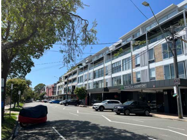
Figure 5 – Residential development along the southern side of Parraween Street (shoptop housing)
