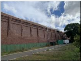
SYDNEY WATER RESERVOIR BRICK WALL
