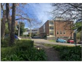
VIEW OF MERRIANG HOSPITAL FROM PARK ACROSS MERRIANG AVENUE SOUTH
