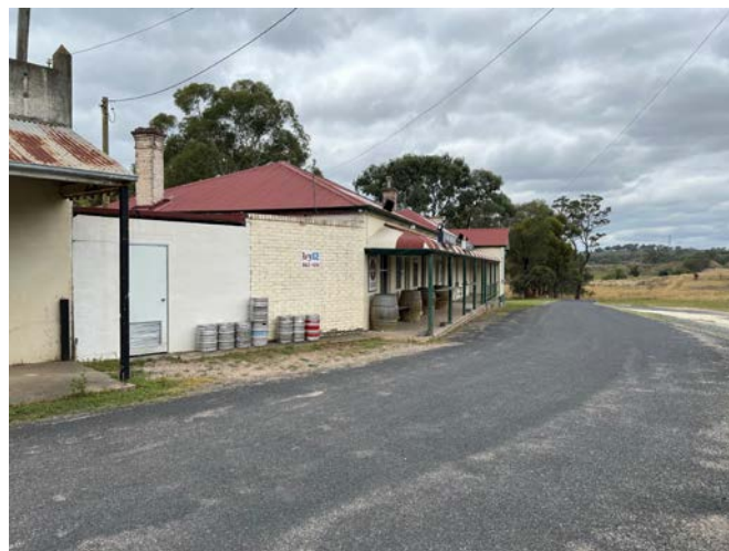
5. View of Lue Hotel from Cox Street
