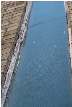
S45 – Rotting of the timber window frames and window cracking at the storage building
