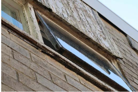
S43 – Rotting of the timber window frames of the storage building
