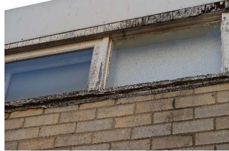
S38- Rotting of the timber window frames of the storage building
