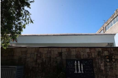
S29 – View of Synagogue roof from Flood St
