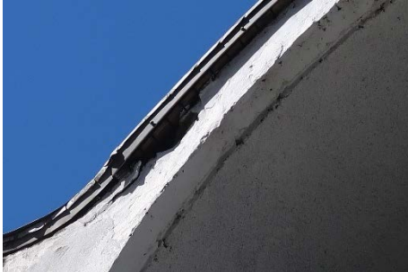
S23 – Significant concrete spalling of the concrete arch at the Northern end
