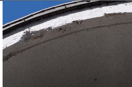
S20 – Significant concrete spalling of the concrete arch at the Northern end
