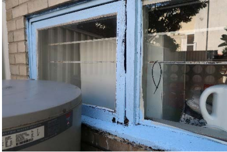
S37 – Rotting of the timber window frames of the storage building
