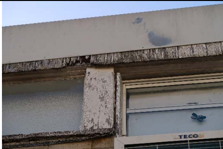
S37 – Rotting of the timber window frames of the storage building
