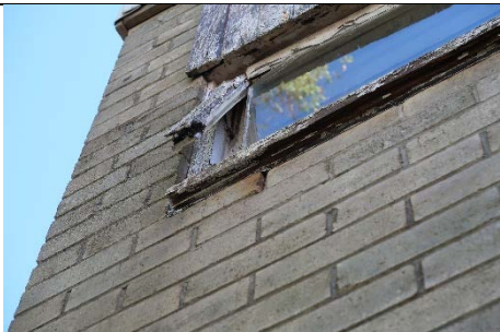
S39 – Rotting of the timber window frames of the storage building
