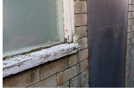
S44- Rotting of the timber window frames of the storage building
