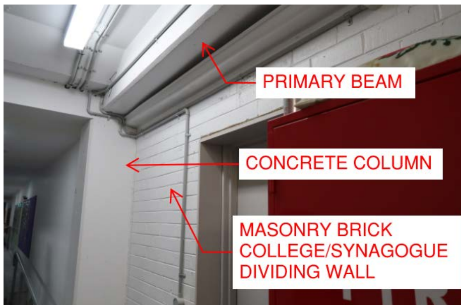
Figure 3 – Building Description Summary (View from College Building)
