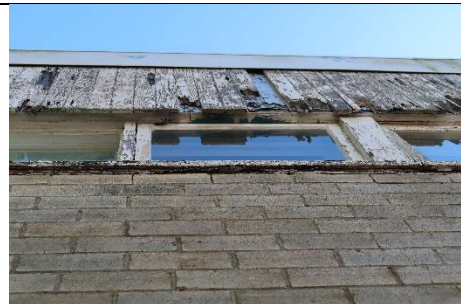
S40 – Rotting of the timber window frames of the storage building
