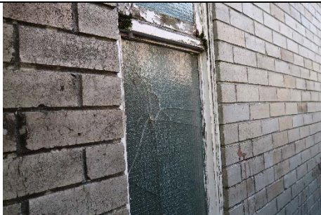
S43 – Rotting of the timber window frames of the storage building
