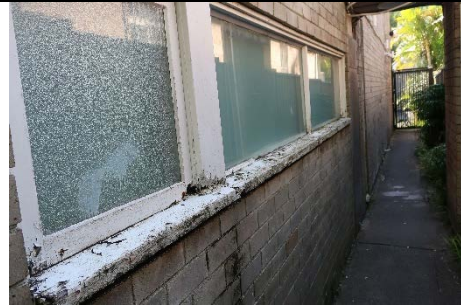
S38- Rotting of the timber window frames of the storage building
