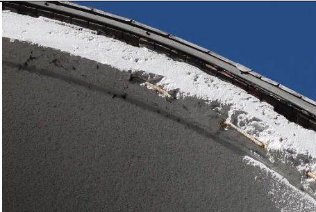
S19 – Corrosion of exposed rebar and concrete spalling of arch at Northern end
