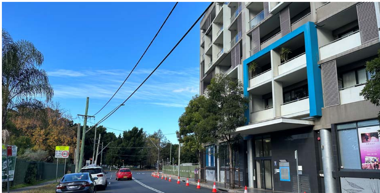
Figure 3 | Hassall St facing east. The site is on the far right marked by green fencing and No.31-37 Hassall St is on the immediate right (Source: DPE, 2023)
