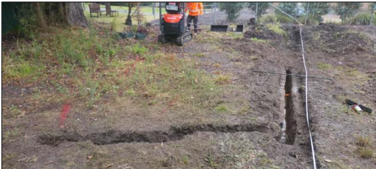
Figure 22 | Root investigations around T1 in line with the basement extent illustrating no significant tree roots (Arterra Consulting Arboriculture 4 July 2023)
