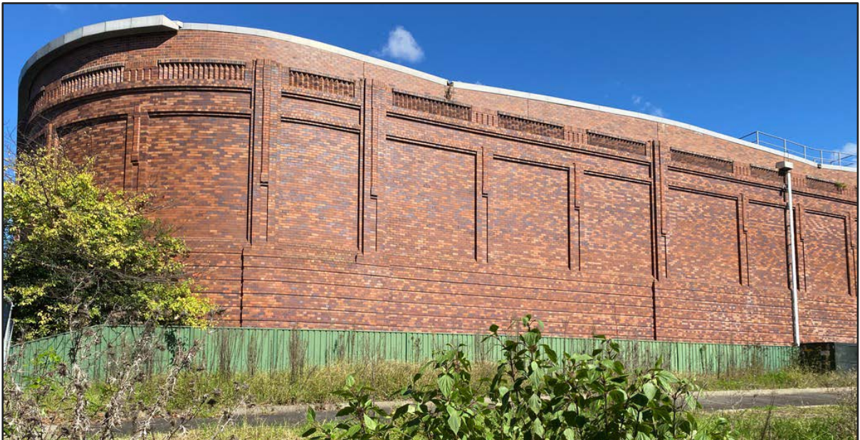
Figure 6 | Sydney Water heritage listed reservoir to the south of the site
