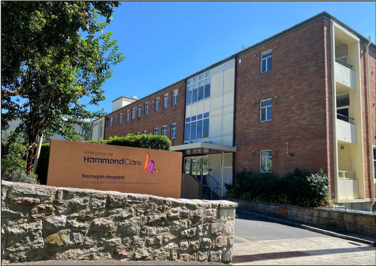
Figure 3 | Existing main entry to Neringah Hospital looking north-west from Neringah Avenue South
