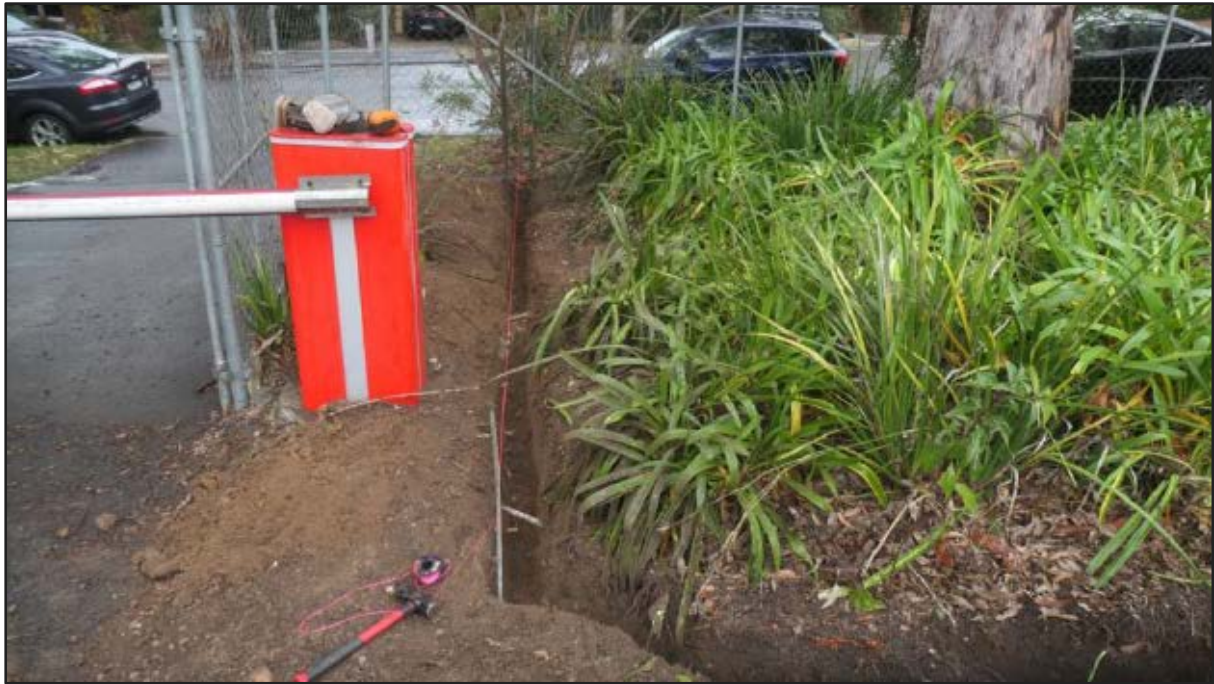
Figure 21 | Root investigations around T32 illustrating no significant tree roots (Arterra Consulting Arboriculture 4 July 2023)
