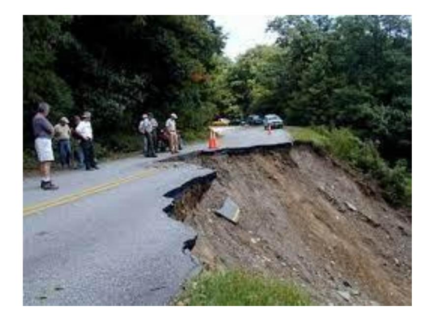
Liquefaction and failure of road Base. Foto:SoilCon archive (SALIVA)
