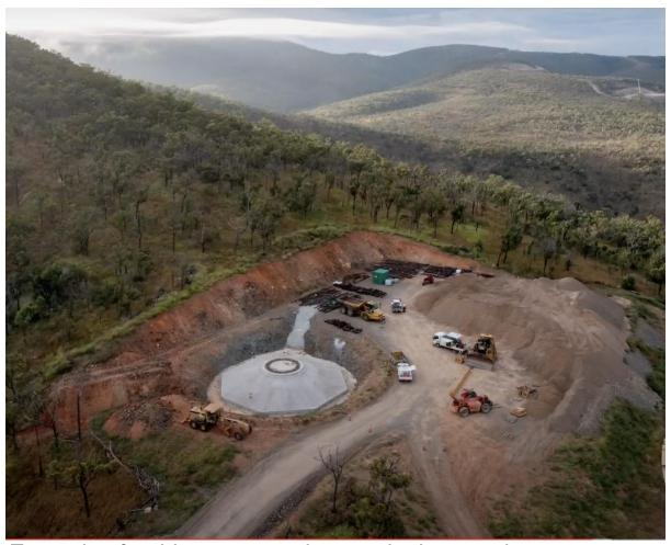
Example of turbine construction on sloping terrain
