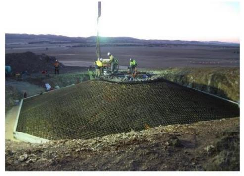
Figure 3-9 Typical Gravity Foundation for a Wind Farm (ENGIE Willogoleche Wind Farm in construction)
