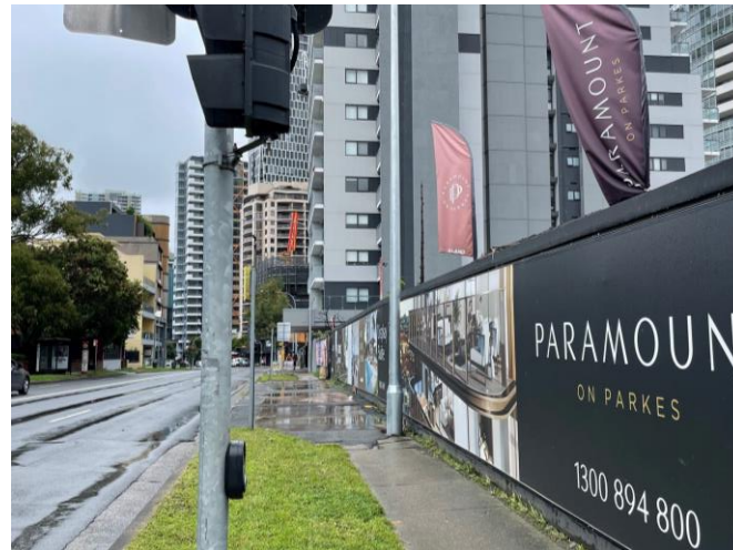
View westward along Parkes Street
