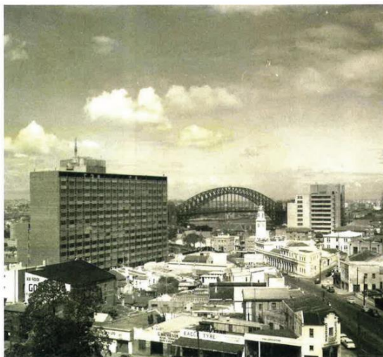
MLC, VIEW FROM NORTH WEST, LATE 1950s
