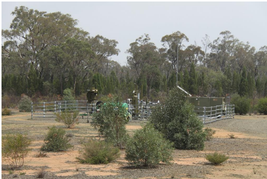
Zooming in on the well site shows trees planted very close to the well
