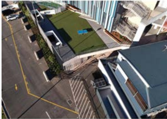
Image 2: SE corner unit of Block A, at sixth floor window. Six metre set back from School boundary (fence line).
