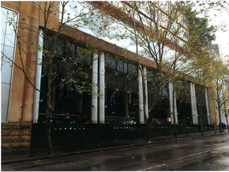
CURRENT VIEW FROM PYRMONT STREET
