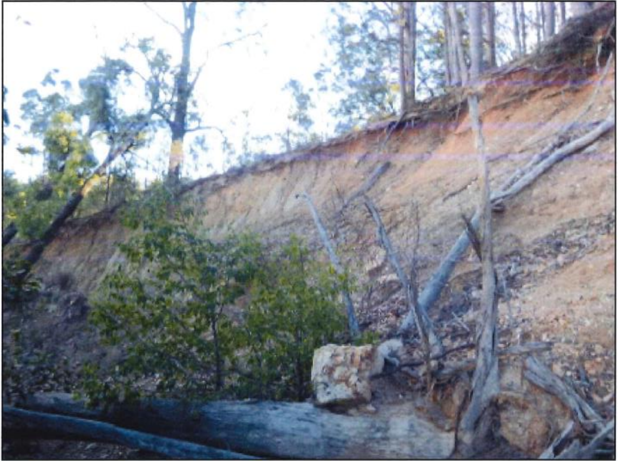
Plate 5: View of an area of previous rehabilitation works that have exacerbated erosion.
