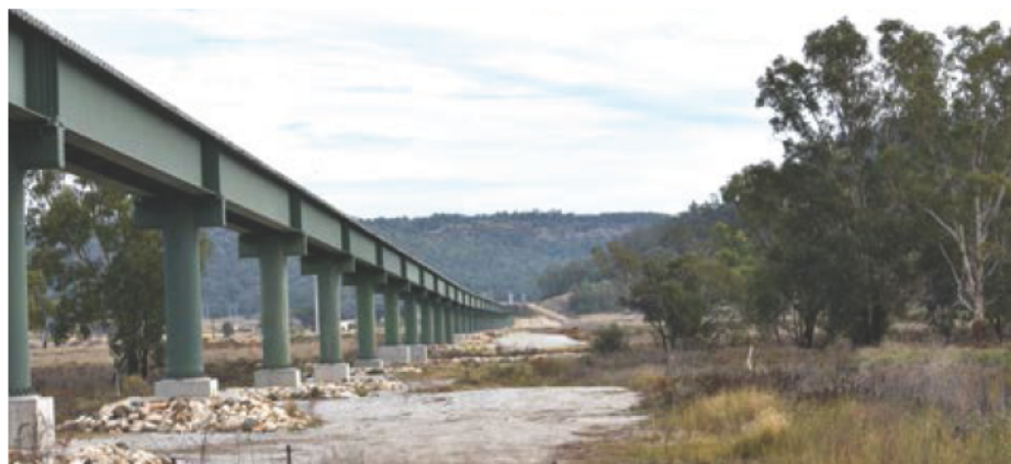
Gins Leap Gap railway viaduct bridge in the Boggabri area crosses at the major constriction in the Upper Namoi Valley on bedrock, which is the safest place to cross. Photo: Ken Crawford.
