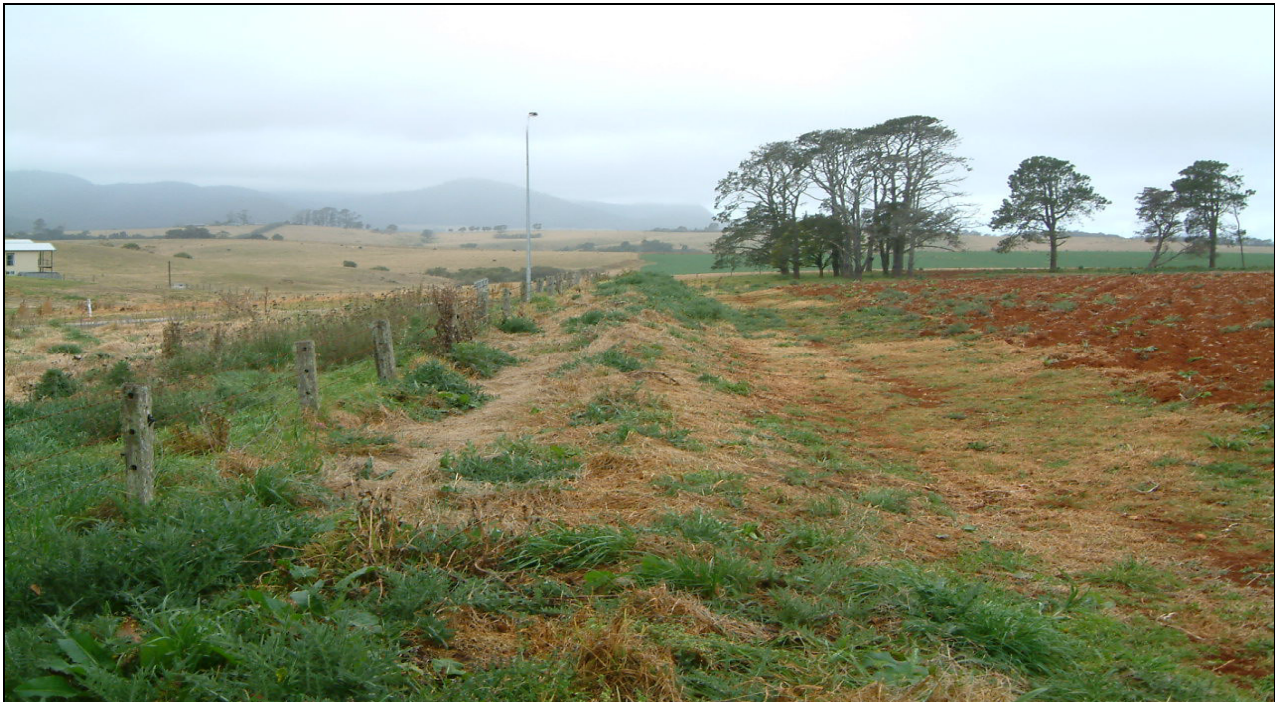
Figure 6-2 Photograph of typical peak diversion bank
