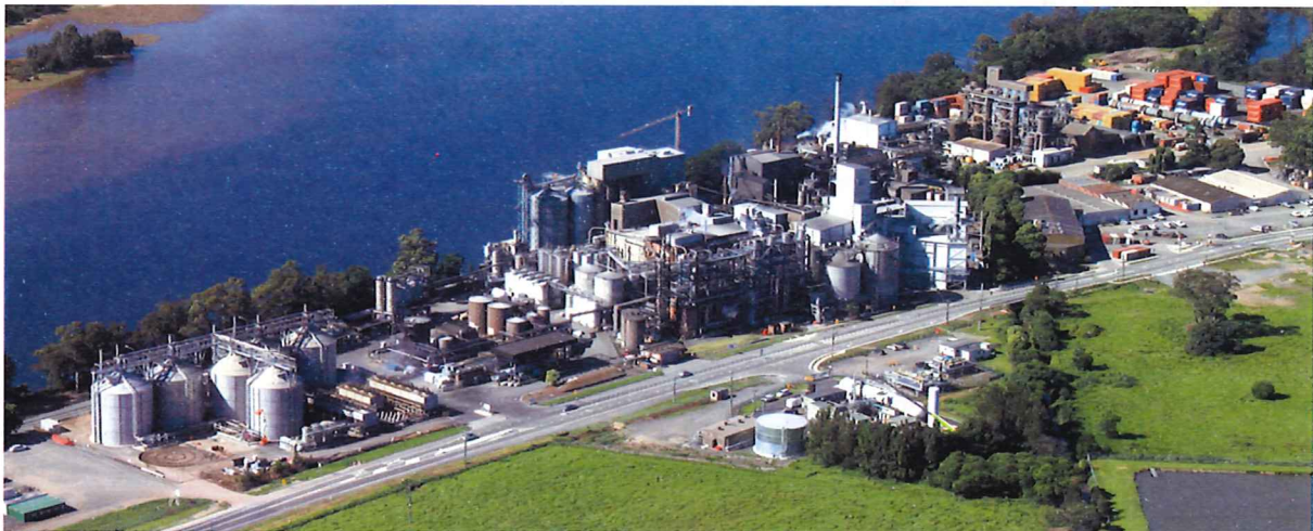
Shoalhaven Starches Factory, Bomaderry
