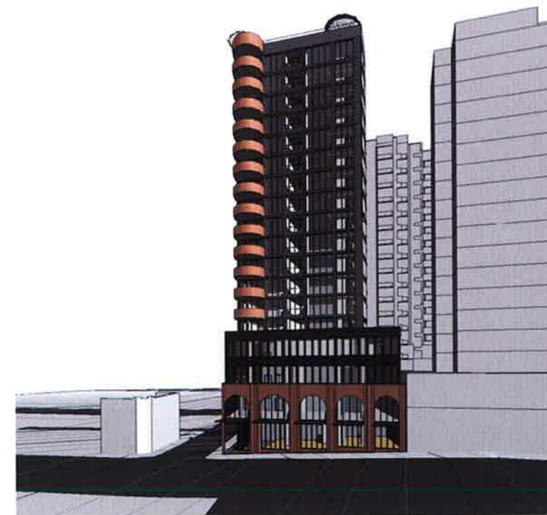
View_Redfern St Looking West
