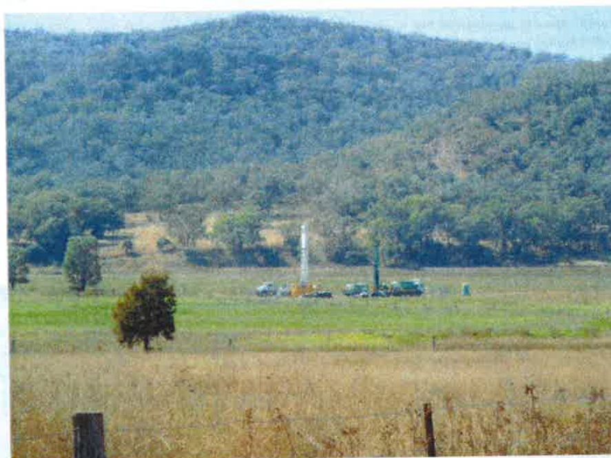
Figure 4-9 Drilling at Test Site 4 adjacent to Bylong River
