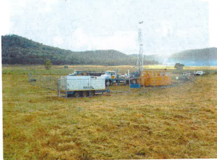
Figure 4-6 Drilling at Test Site 1
