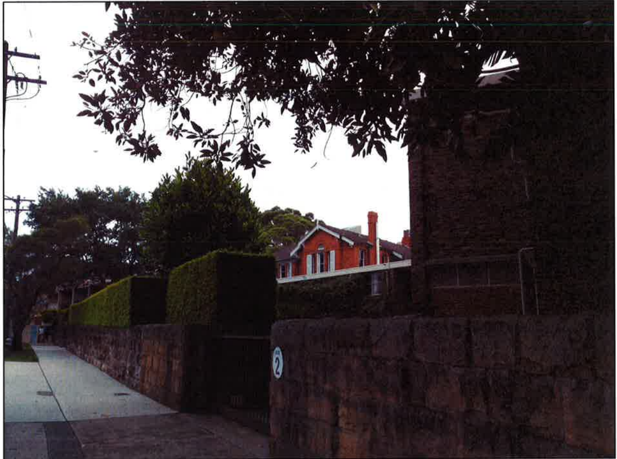
Figure 4: View of the site along Albion Street (from Gate 2 towards St Johns Building)
