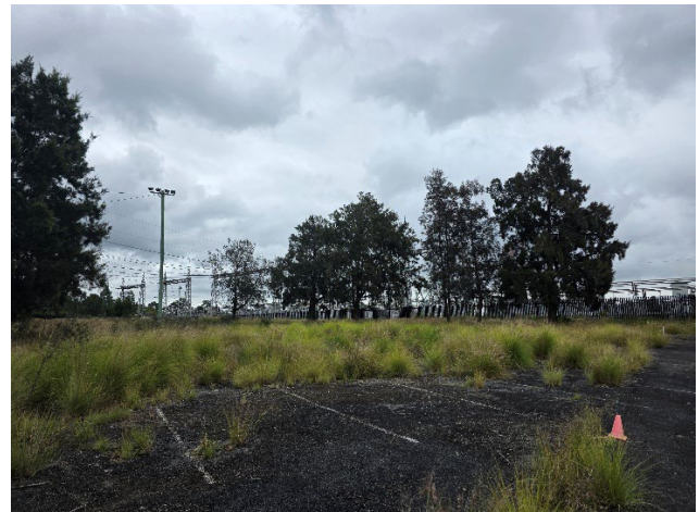
Figure 4 – hardstand in foreground with existing substation in background
