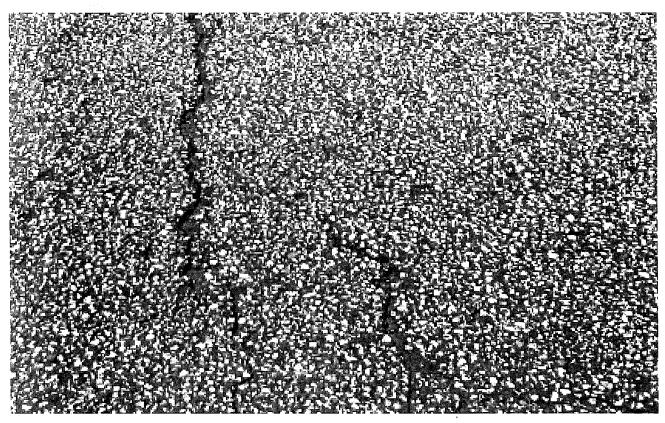
Photograph 6: Close up of the lighter coloured pavement, showing light coloured rhyolite aggregate
