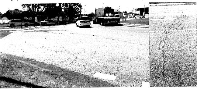
Photograph 8: Rhyolite roundabout at Tighes Hill 3-2-2021 in poor condition.
