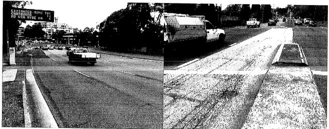
ph 16: Rhyolite intersection Pacific Hwy A1, Pymble in poor condition and a Rhyolite turning lane, Warringah Road Forestville in poor condition (24-6-2021). Photograph 16:
