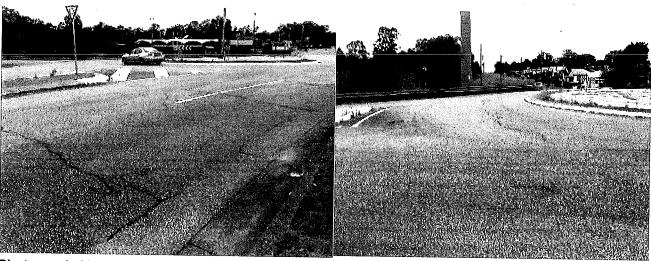
Photograph 10: Rhyolite roundabouts on Victoria Street and Northcote Street, Kurri Kurri in poor or deteriorating conditions on 16-3-2021.
