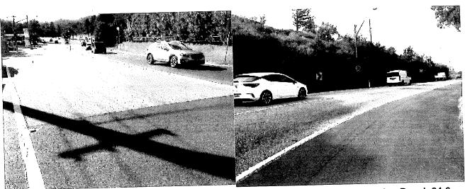
Photograph 17: Rhyolite in traffic lights breaking area Barrenjoey Road, Avalon Beach 24-6-2021 in good condition. and on bends Barrenjoey Road, Bilgola Beach 24-6-2021 in reasonable condition.
