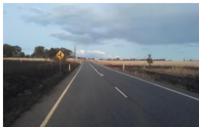
Fire jumped road from left to right
