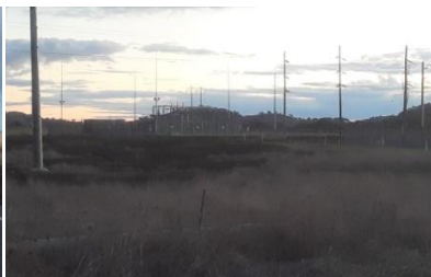
Fire reached solar works fence
