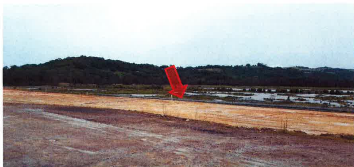
Figure 11: Existing Fence adjacent to saltmarsh rehabilitation area
