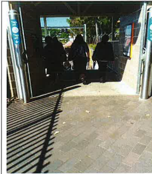
The entrance/exit from Cornwallis St to Platform 10. This thoroughfare is 2.3 metres wide.
