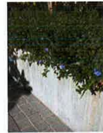
INSITU CONCRETE PLANTERS
