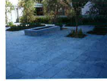
STACKBOND GRANITE PAVING
