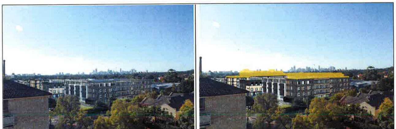
Figure 13: Approved (left) and proposed (right) north west view from the balcony of 5/125 King Street
