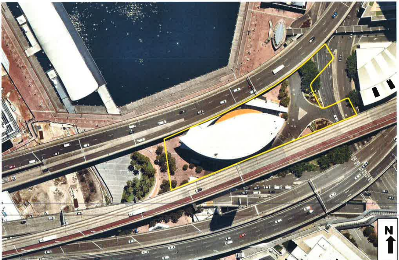
Figure 2: Aerial photo of the site showing the approximate "ribbon" building footprint including air space over Harbour Street (yellow line)
