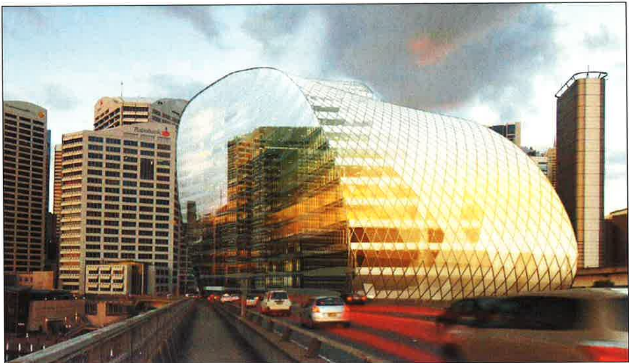
Figure 12: The northern and eastern elevations and roof as seen from the Western Distributor (Source: Hassell Urban Design Report)
