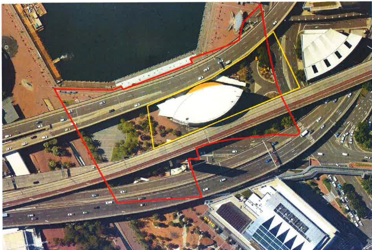
Figure 1: Aerial photo of the site showing the total zone of influence site area in red and the approximate tower building footprint in yellow (Base Image Source: Nearmap, 2014)
