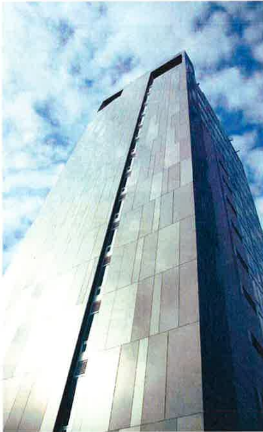
CC1 - Tower Walls
