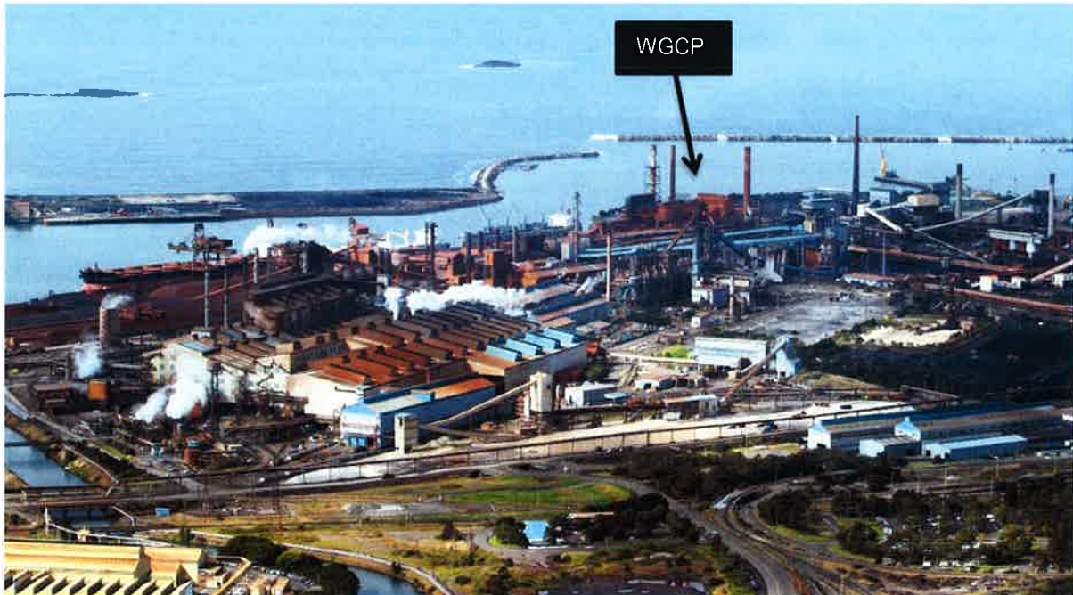
Figure 2: Extensive steel making infrastructure at the Port Kembla steelworks
